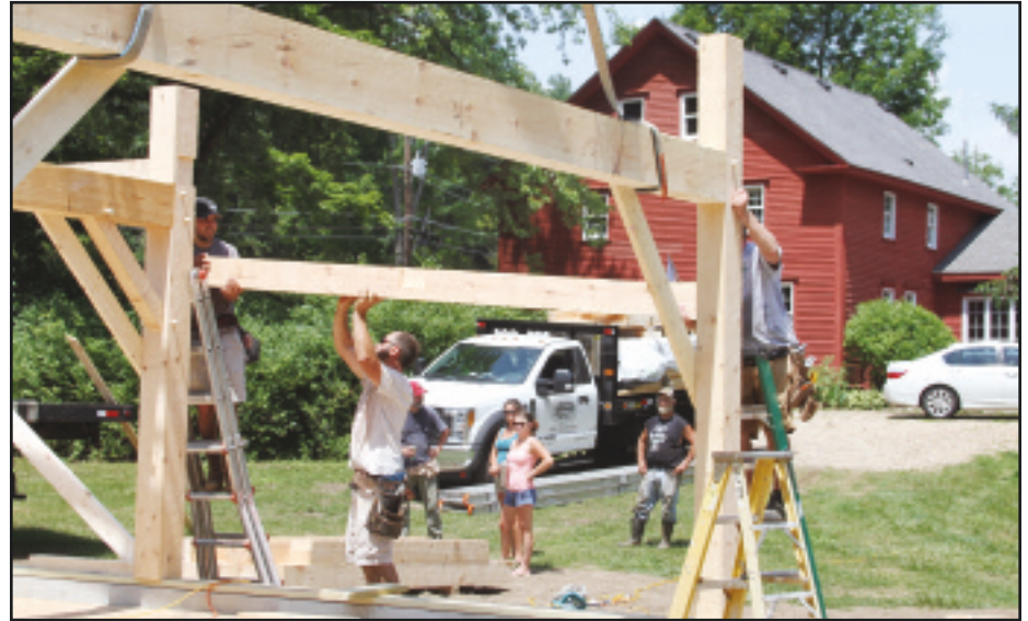
Crews worked during a hot and humid day last week to get the post and beam barn frame up in Hampstead for a new Sugar Shack. Photo by Chris Paul
