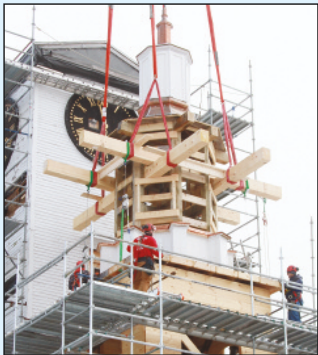
The crew from Preservation Timberframing Inc. carefully fastened, hoisted and placed the massive Steeple onto the bell tower last week as the First Parish Churches preservation efforts continued. Once the finish work is done on the 60 foot structure it will be lifted into its original spot. The church hopes to be done during the Nutfield 300th Anniversary celebration. Photos by Chris Paul
