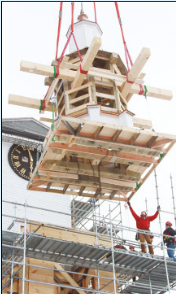
The crew from Preservation Timberframing Inc. carefully fastened, hoisted and placed the massive Steeple onto the bell tower last week as the First Parish Churches preservation efforts continued. Once the finish work is done on the 60 foot structure it will be lifted into its original spot. The church hopes to be done during the Nutfield 300th Anniversary celebration. Photos by Chris Paul
