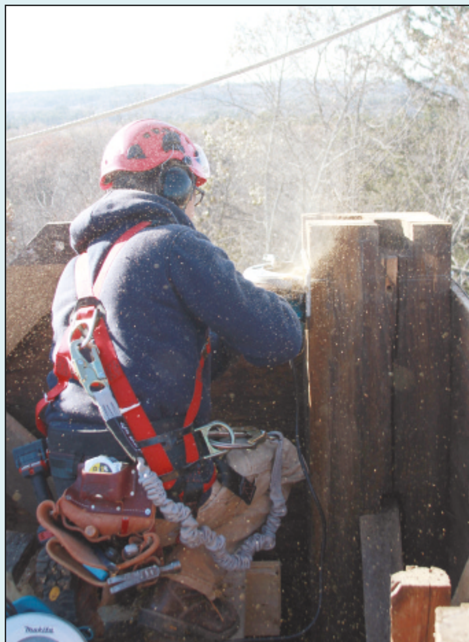
Zachariah Whitridge, one of the Preservation Timber Framing Inc. construction workers has a great view of East Derry while he prepares a beam on the First Parish Church Meetinghouse above the clock to receive the top plate on which the steeple will be placed in the future.
