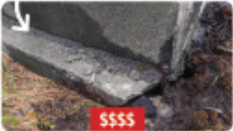
Foundation Damage+Erosion
