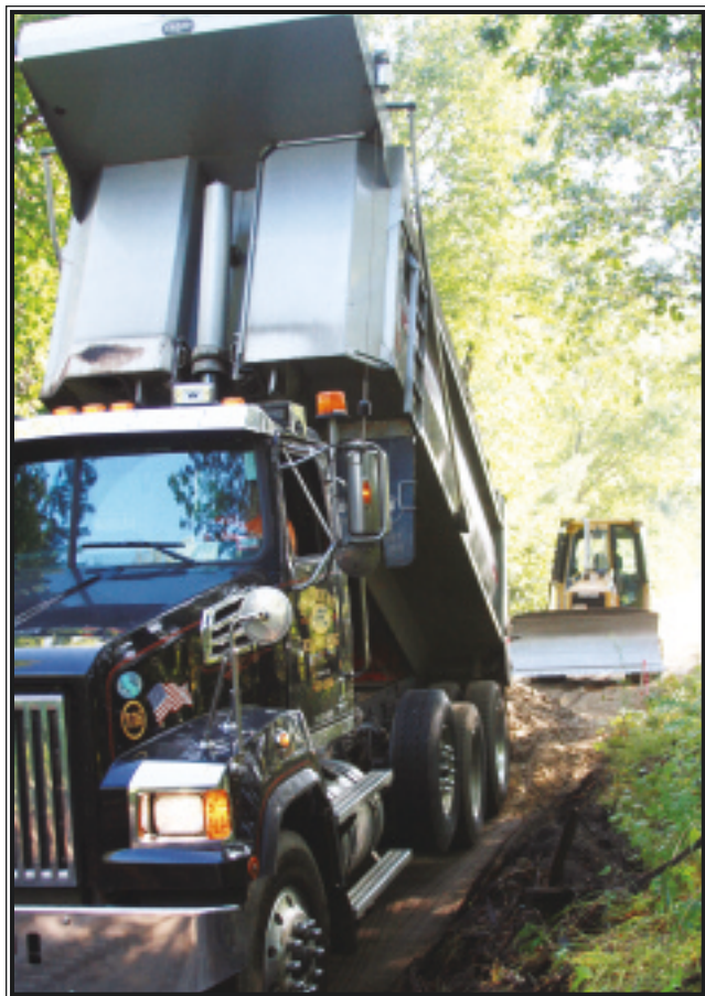
Tons of gravel was being layed on the Rail Trail that will connect Mammoth Road and the Airport.
