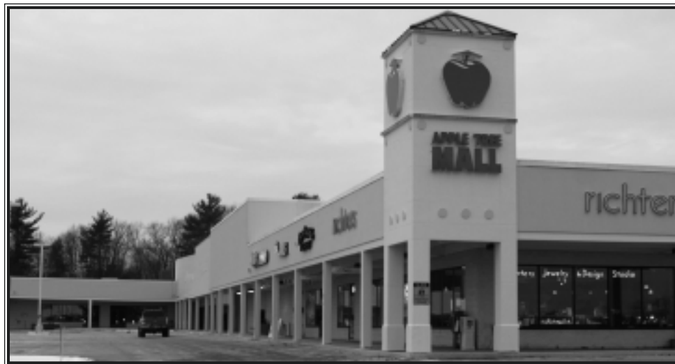
The Appletree Mall is scheduled to be auctioned off on Jan. 27 at 1 p.m. according to St. Jean Auctions of Epping. Photo by Chris Paul
